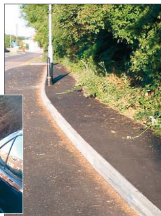
Brook Road Industrial Estate – Parking Improvements
